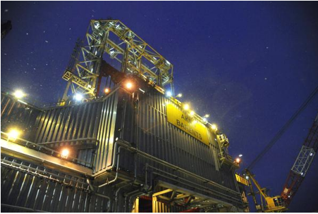
The Aker-Barents drilling rig in the Barents Sea. Photo: Harald Pettersen -Statoil
