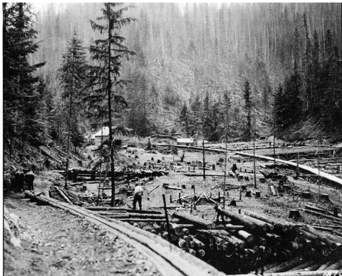
Winton Logging camp on the Skookum Creek sale. In the foreground men are rolling logs into the chute. Horses were used to move the logs along. The flume on the right cost $9,000. Coeur d'Alene National Forest, 1924. Log-1-10
